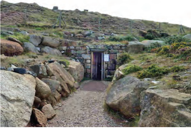
The walk-in entrance to Wheal Mexico, rediscovered in 1995 after removal of waste in preparation for the heritage site at Geevor. Photo Casper Tilly
